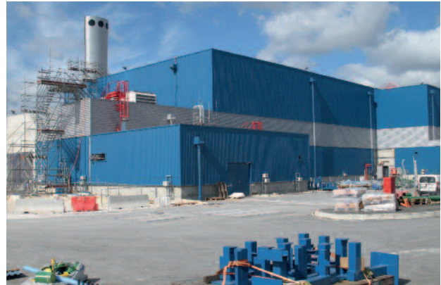
External view of the REC II facility under construction at the GEORGES BESSE II plant – October 2011
