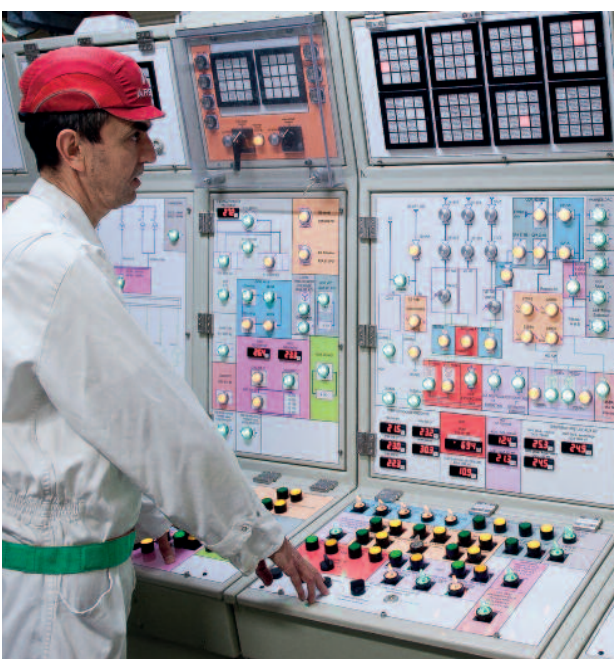
Backup control panel in the MELOX plant. The “utilities” operations supervisor supervises the periodic inspections and tests
