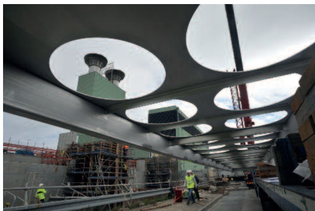
Construction site of the glass storage building extension on the La Hague site (EEVLH)
