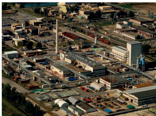
The COMURHEX plant at Tricastin
