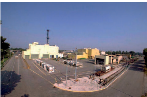
The TU5 facility on the Tricastin site
