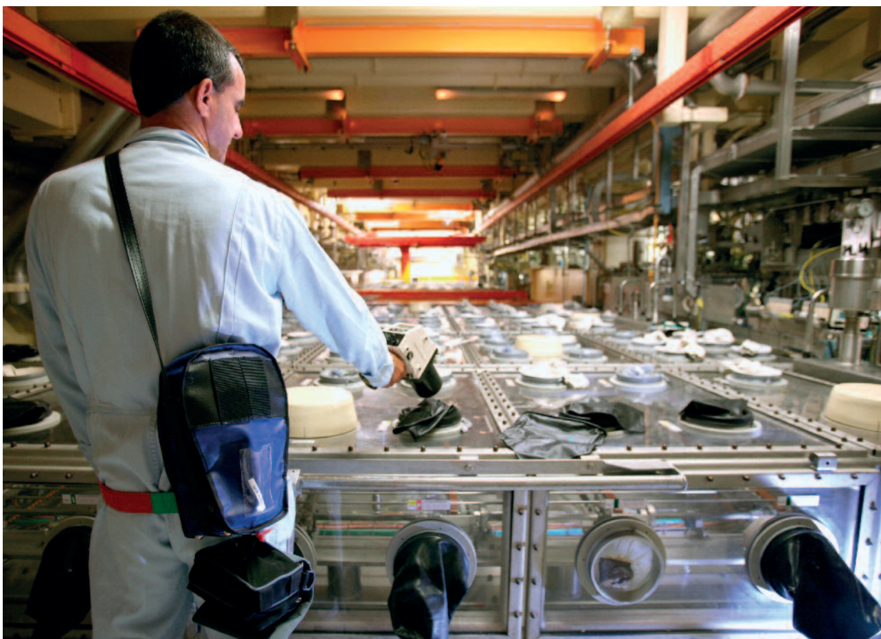
Radiation protection inspection on the glove boxes in the cladding room in the MOX fuel manufacturing plant at Bagnols-sur-Cèze
